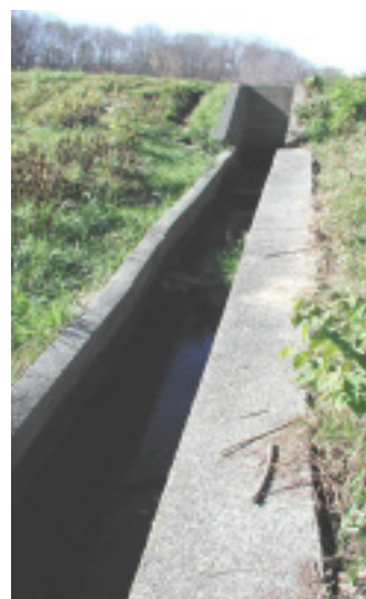
Fishway exit at Shad Factory Pond
