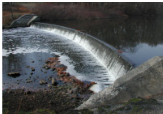
Ten Mile River State Park Dam
