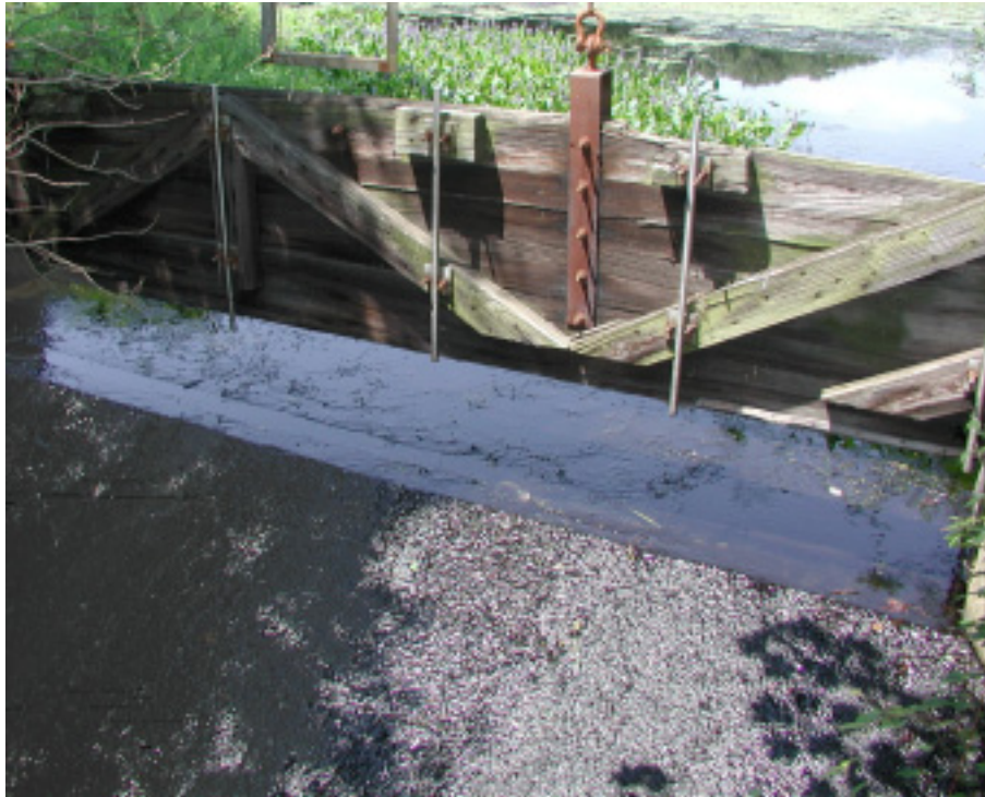
Swan Finishing Dam
