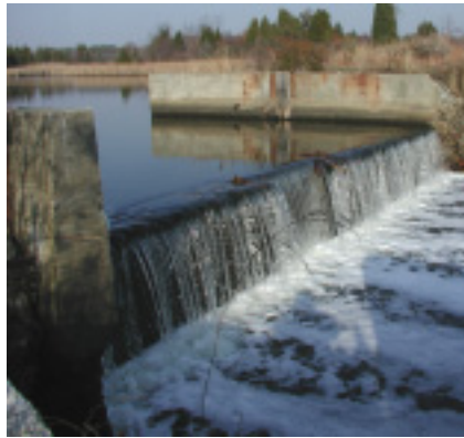
Dam on Mobil Corporation property
