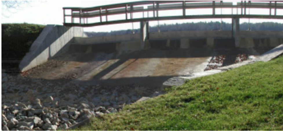
Upper Warren Reservoir Dam
