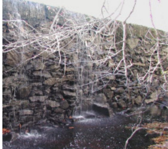
Spillway of Milford Pond Dam, seen from below
