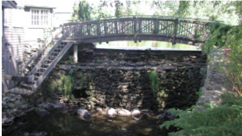
Old Grist Mill Pond Dam
