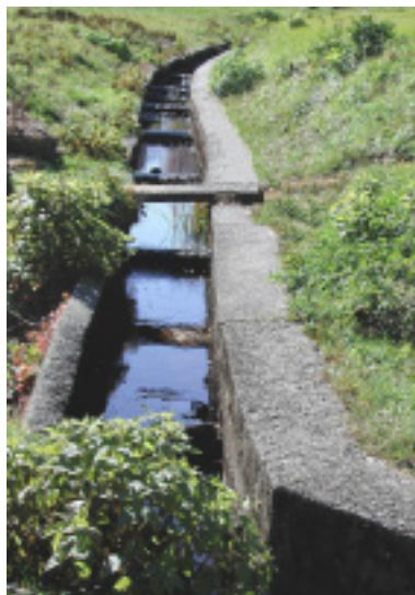
Lower Section of Ladder at Shad Factory Pond
