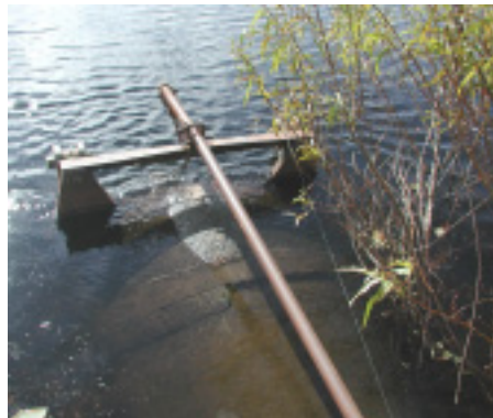
Unnamed Bristol County Water Supply Dam
