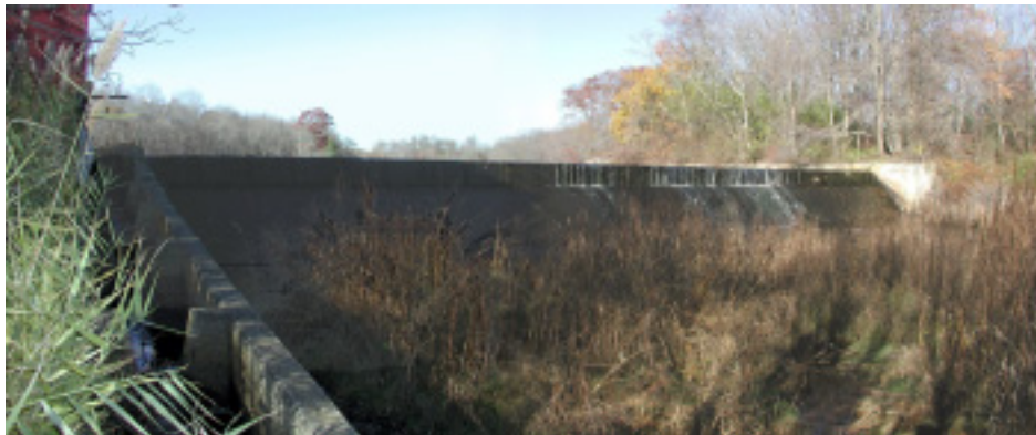
Cole Fishway Dam (with ladder along left side of spillway)
