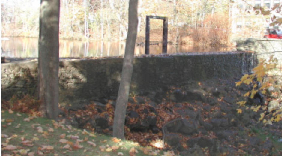
Lewin Brook Pond Dam
